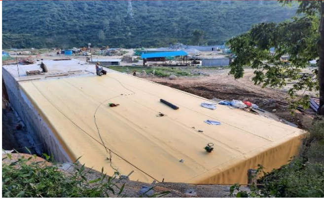
Waterproofing services of rooftop at Arunachal Pradesh
