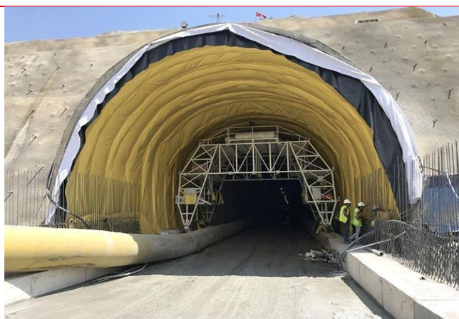
Waterproofing services of tunnel at Maharashtra
