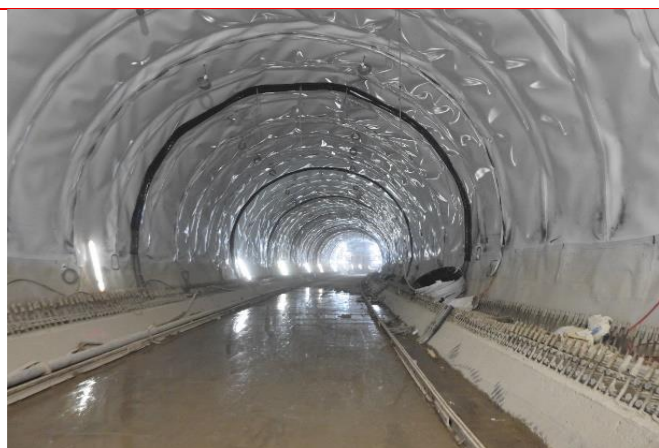
Waterproofing services of tunnel at Himachal Pradesh
