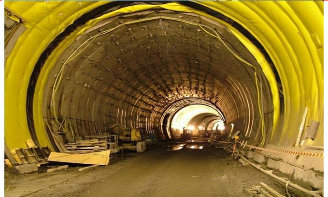
Waterproofing services of tunnel at Odisha
