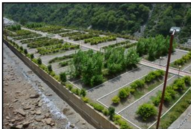
Soil Biotechnology-based STP at Devprayag
