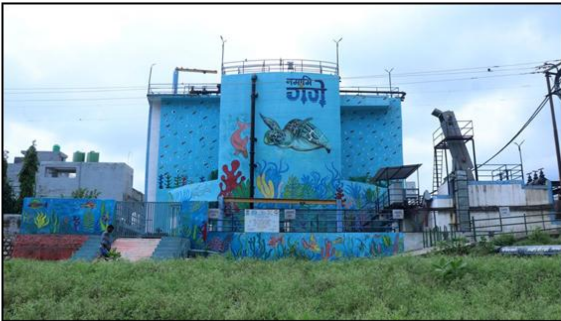
Multi-Storey Sewage Treatment Plant at Muni Ki Reti
