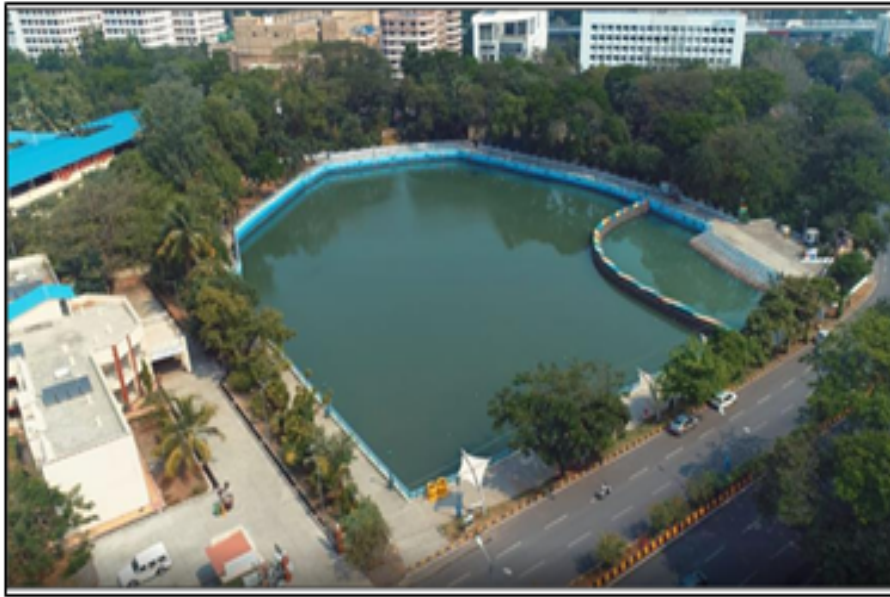
Sewage Treatment in Navi Mumbai
