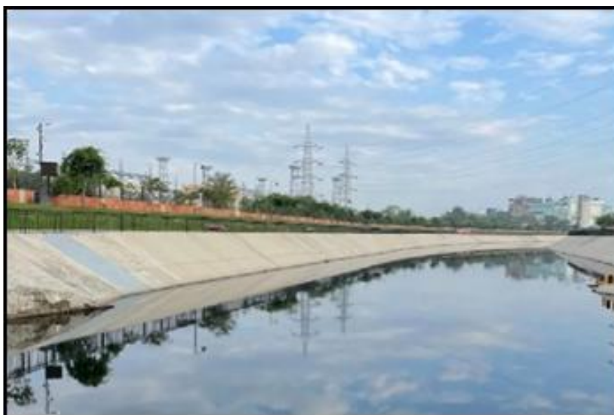
The plant discharging treated water into the Dravyavati River
