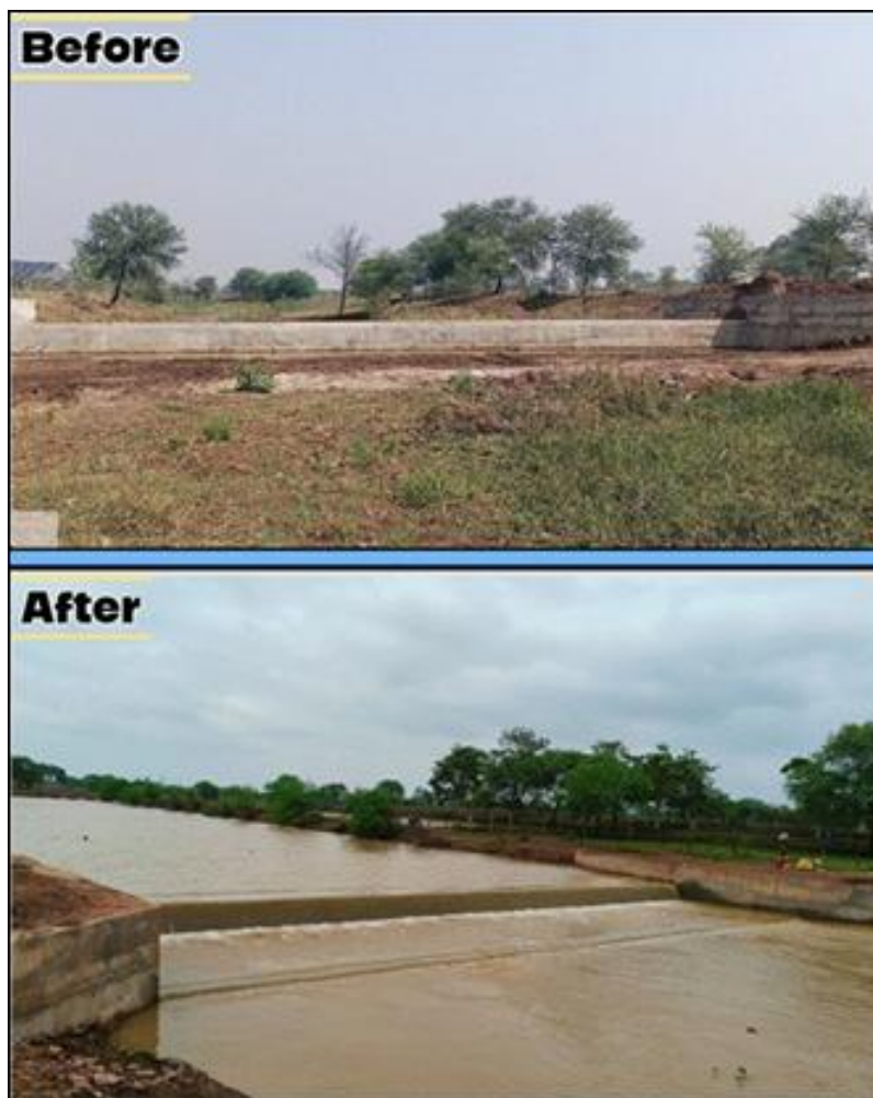
Check Dam in Balod District, Chhattisgarh
