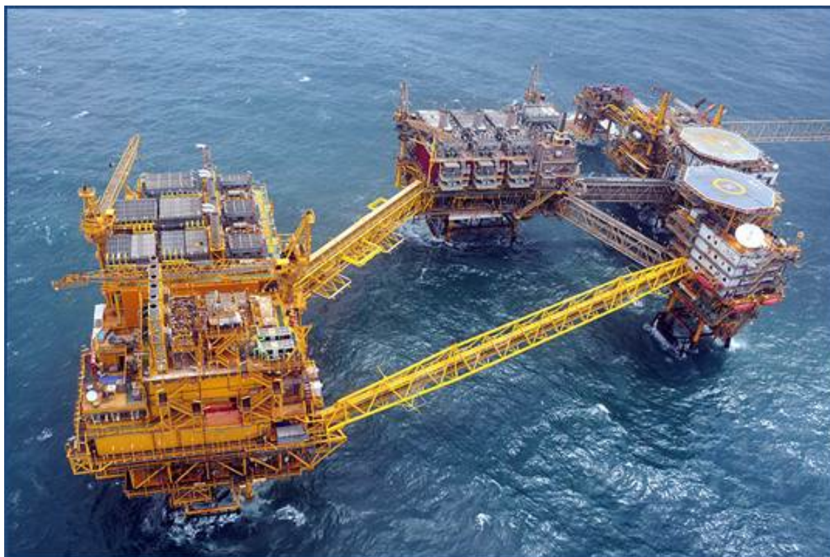
ONGC's Fixed Offshore Platform
