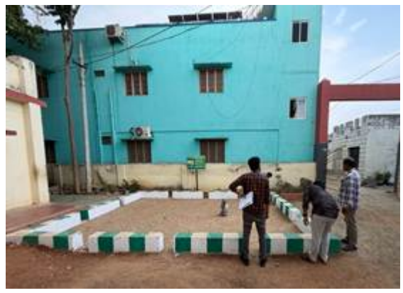
Recharge pits with injection bore wells constructed in Burdwan, West Bengal and Vizianagaram, Andhra Pradesh
