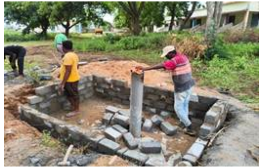
Recharge structures under construction before monsoon in Korba, Chhattisgarh and Warangal, Telanga
