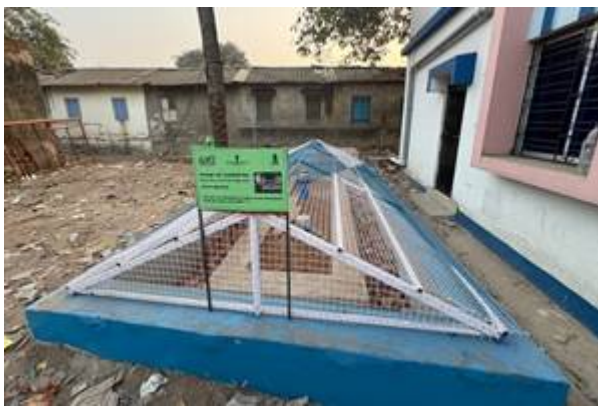
Recharge pits with injection bore wells constructed in Burdwan, West Bengal and Vizianagaram, Andhra Pradesh
