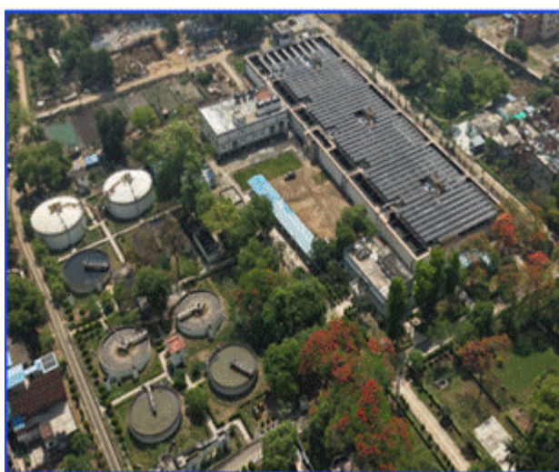
Bhagwanpura, Varanasi - 55 MLD
