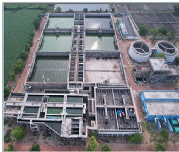
Trial testing commenced on 100 MLD Dhandhupura STP at Agra
