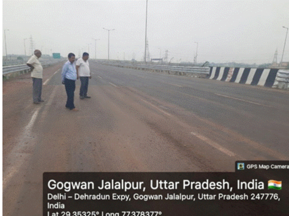
Km 55 after restoration — Gogwan Jalalpur, Delhi–Dehradun Expressway
