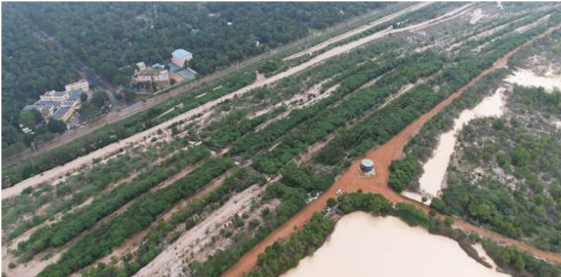
View of External Dump Slope after vegetation growth.
