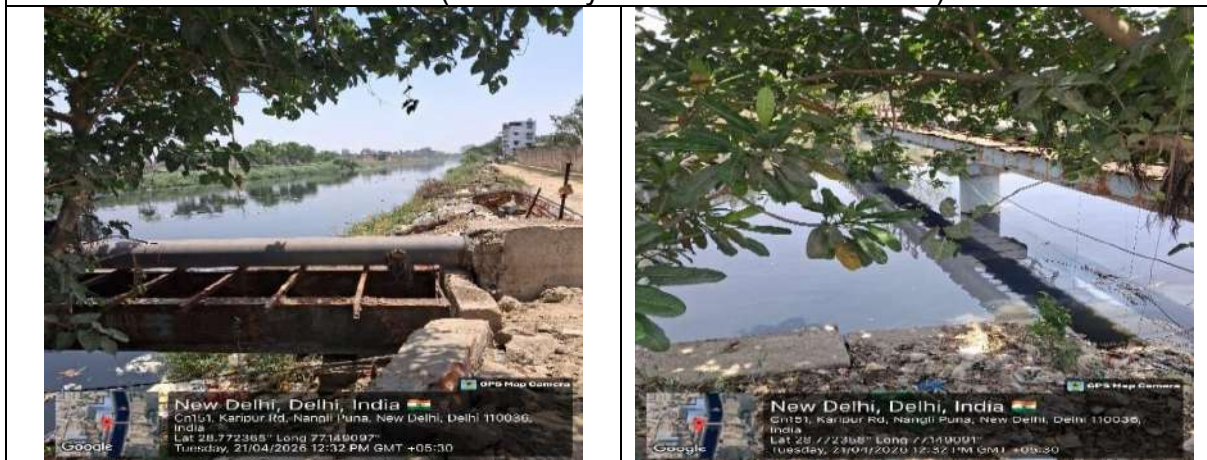
New Drain (AB7) A/C of Alipur Link Drain and Drain No.6
