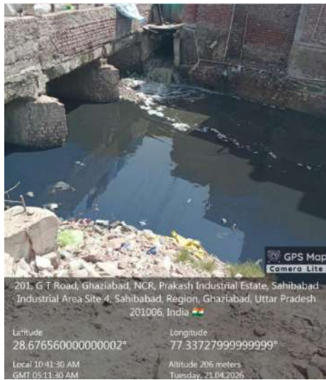
Sahibabad drain near Shaheed Nagar metro station at GT Road
