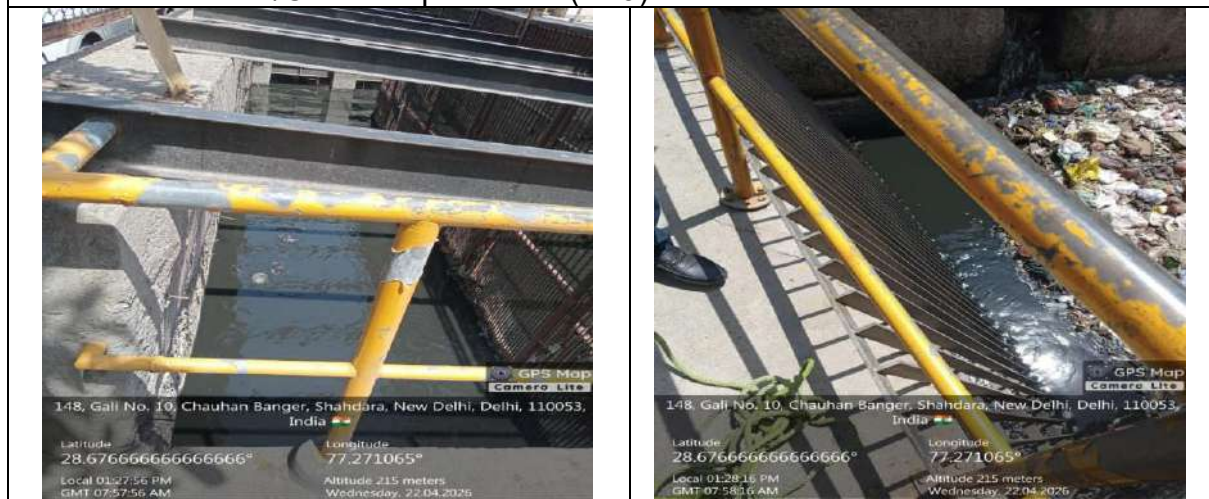
Brahampuri drain (Gokalpur Drain) near Brahampuri drain SPS
