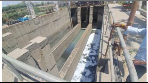
Pankha Road Drain (NB7)
