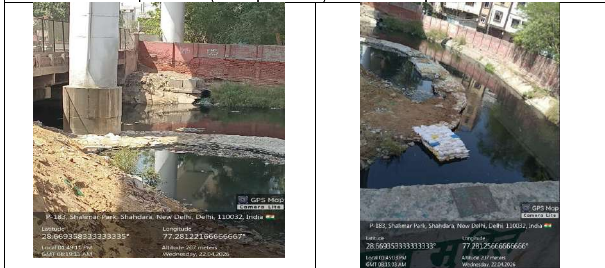
Trunk drain No. 1 A/C of GT Road drain
