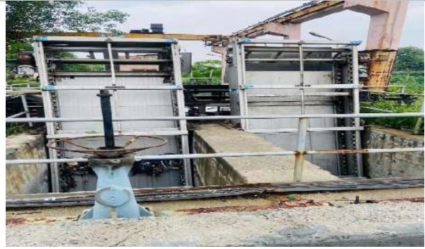
Non-functional (bypass) Also, bar screens choked with solid waste
