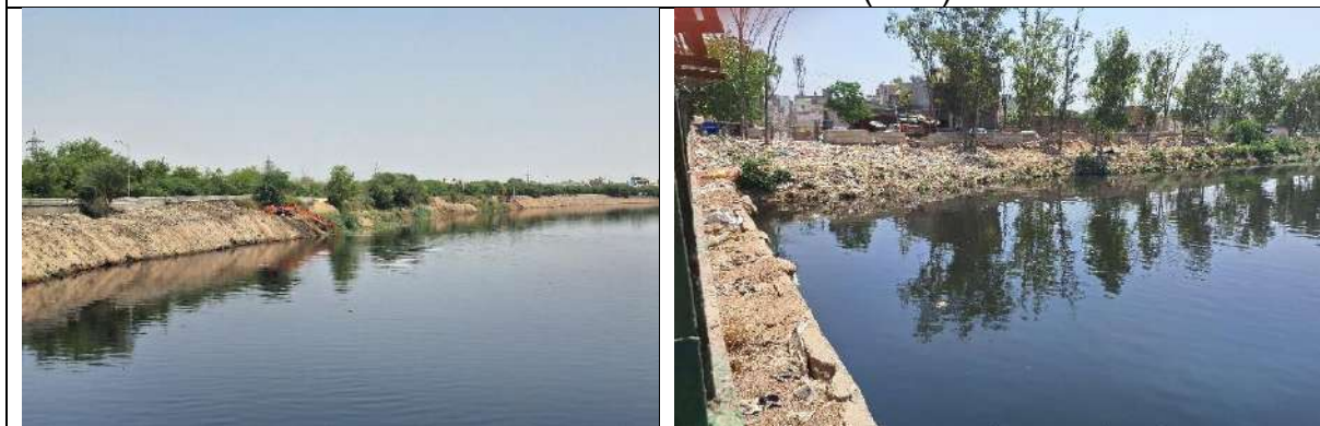
Sahibi river A/C of Mungeshpur drain
