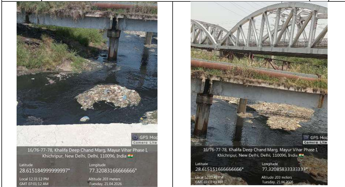
Ghazipur drain A/C of Vinod nagar drain
