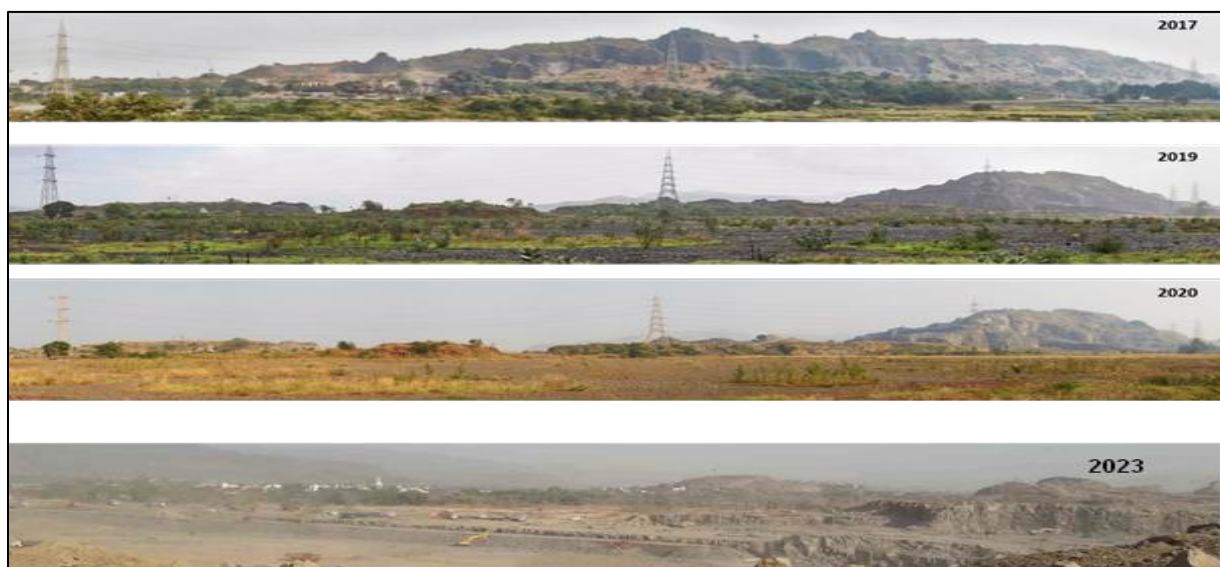
Figure 6: Ulwe Hill Cutting at NMIA site - Progressive Developments
