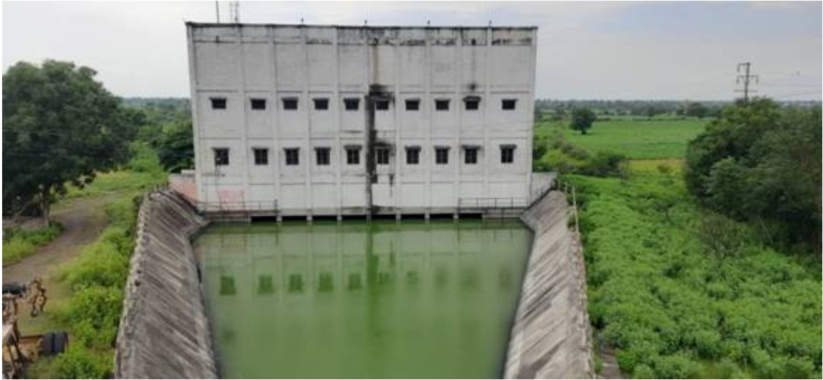
Dehani LIS Pump House
