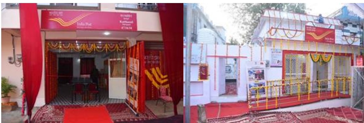
Renovated Post Office Buildings at Katthamil & Kolaras in Madhya Pradesh
