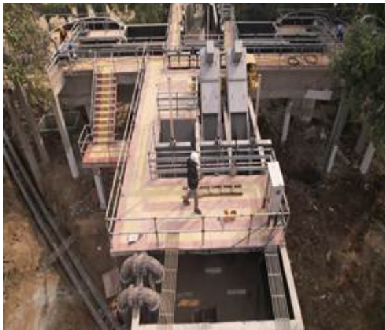
55 MLD STP at Assi BHU, Varanasi
