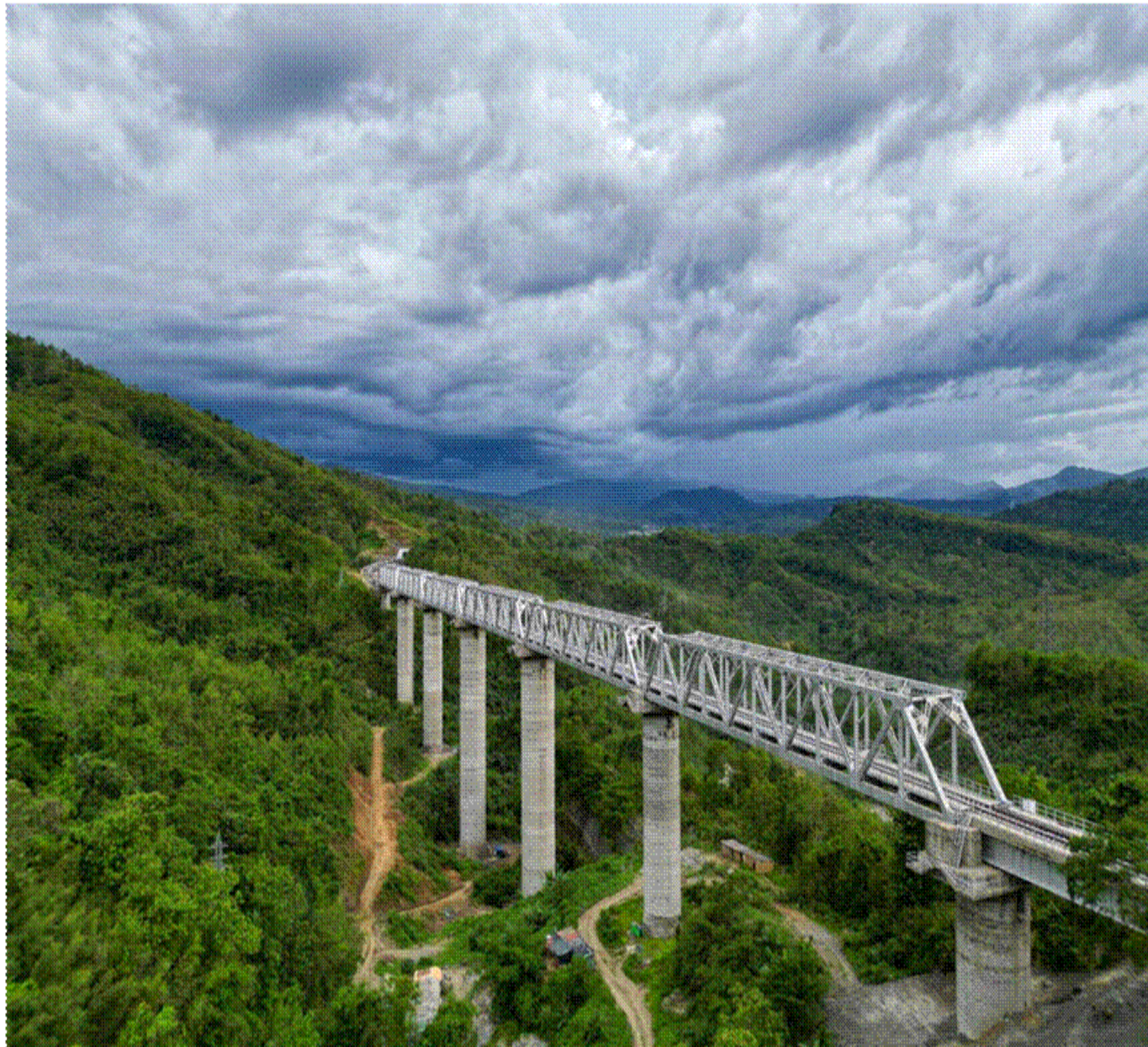
Bridge No. 144 (42 metre taller than Qutub Minar) of Bairabi-Sairang Rail Line
