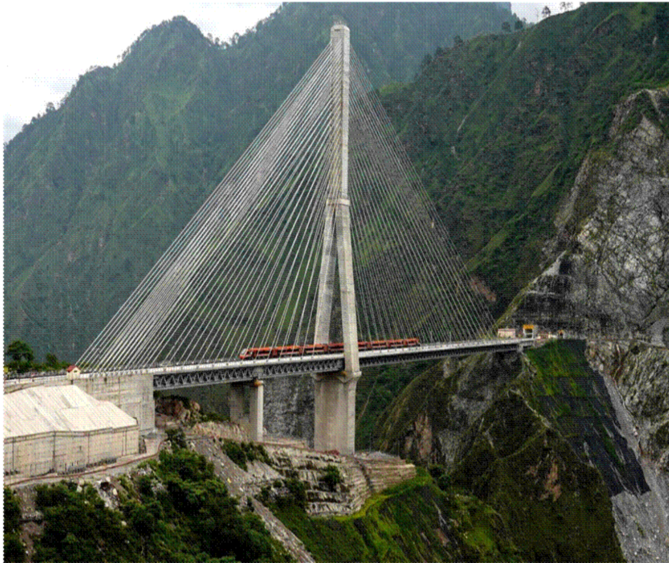
Anji Rail Bridge
