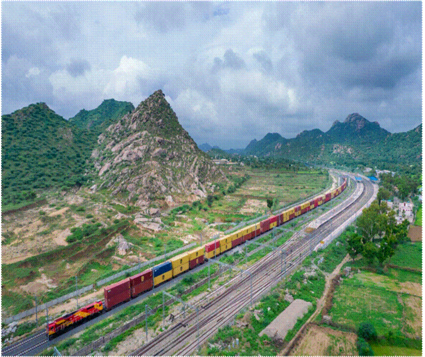
Dedicated Freight Corridor
