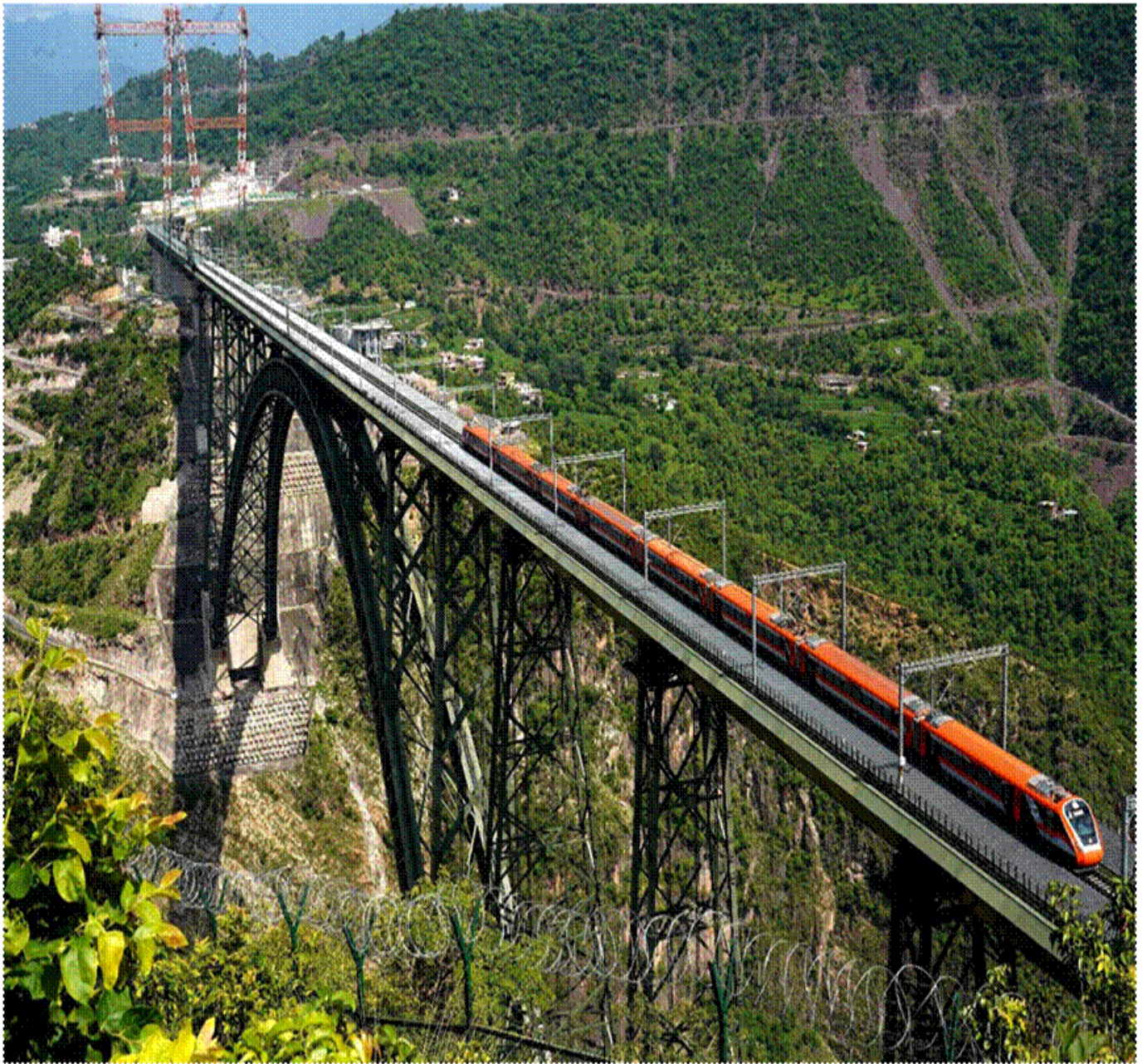
Chenab Rail Bridge
