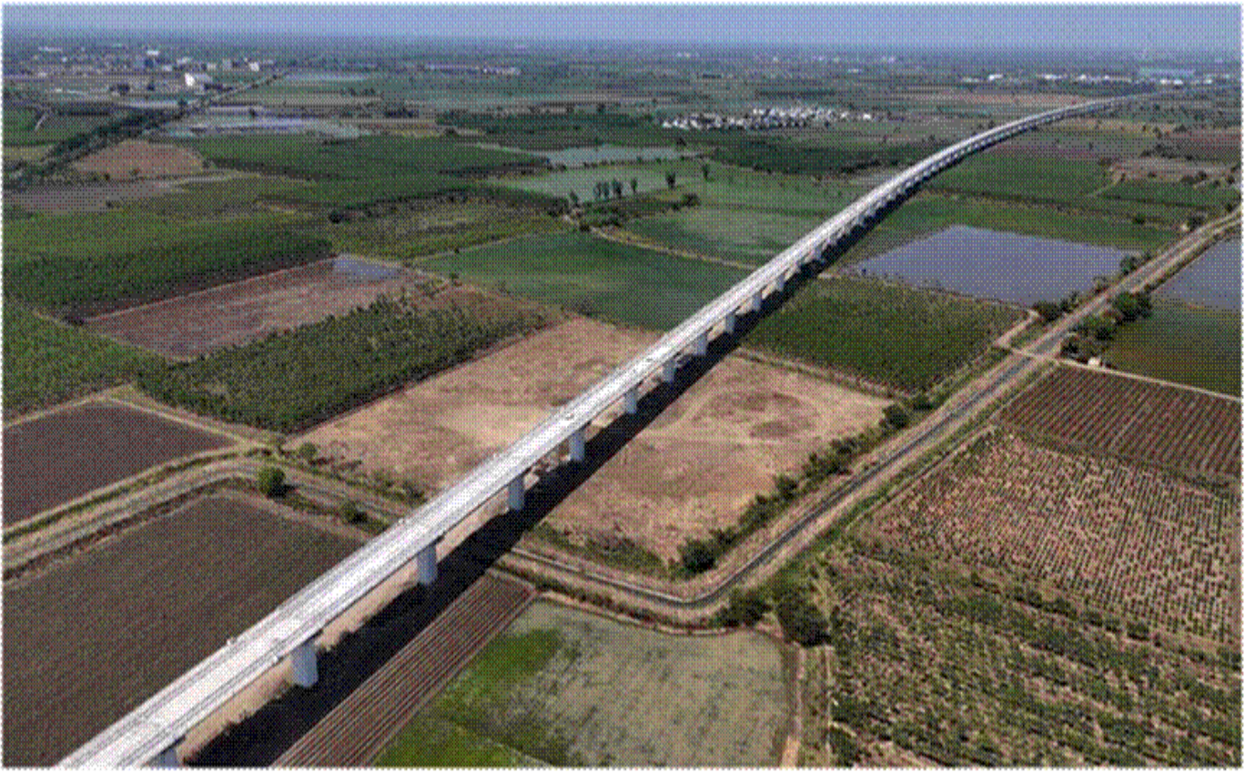
Viaduct in Surat district, part of the Mumbai-Ahmedabad Bullet Train project
