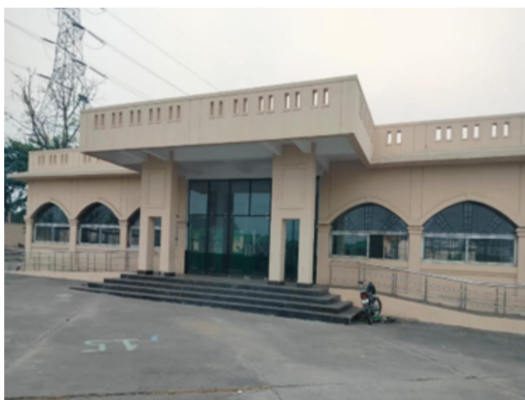
Construction of associated infrastructure in Nagpur city under PM-eBus Sewa Scheme
