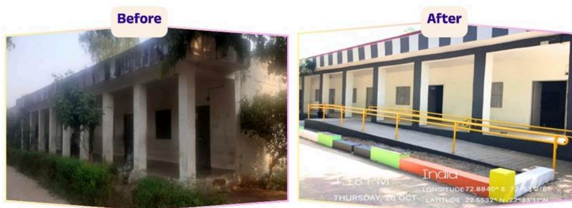
VALASAN PRIMARY SCHOOL, GUJARAT
