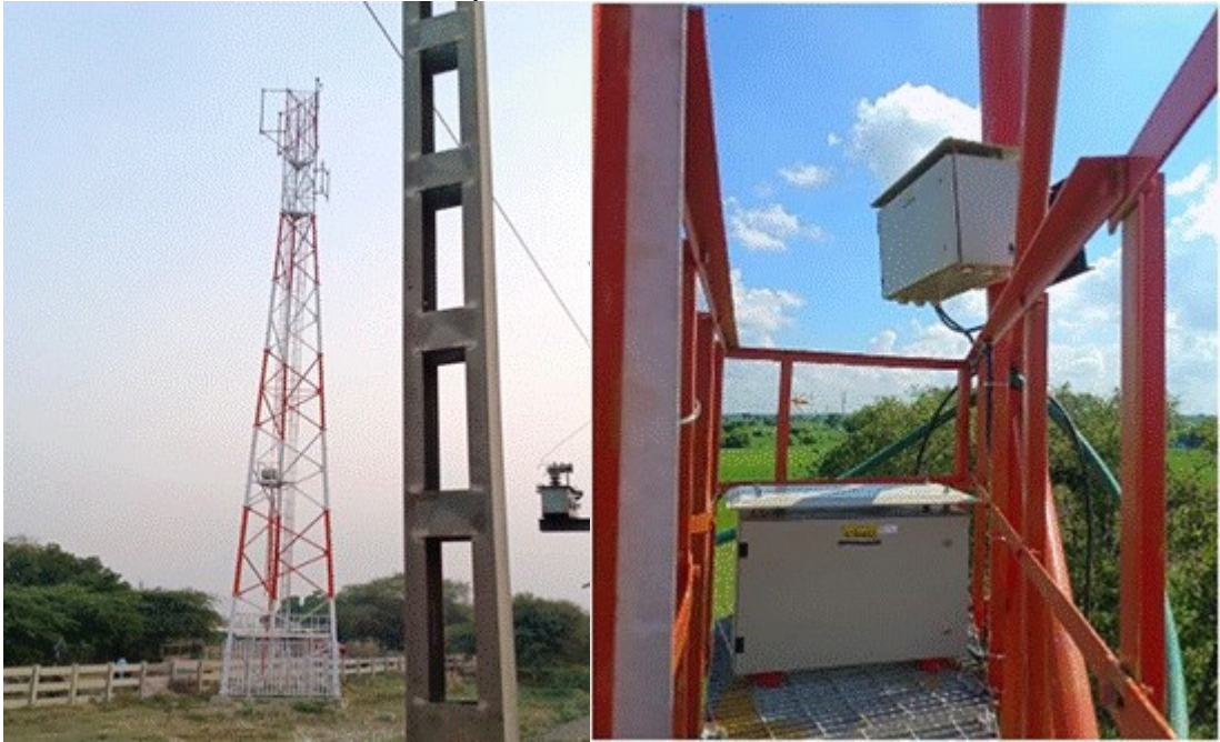
(Telecom towers installed)
