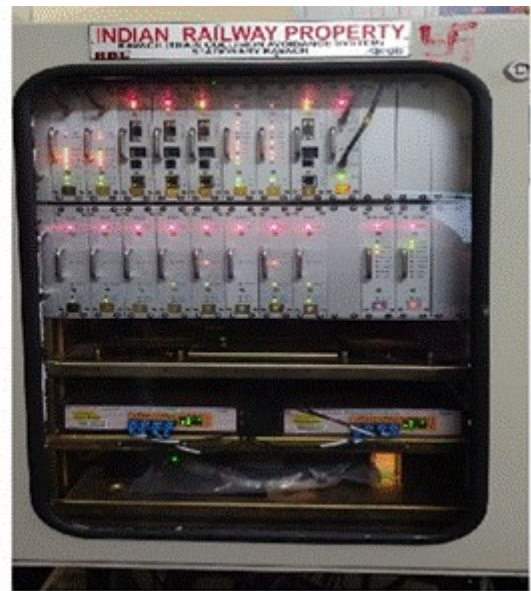
(Installation of Station Kavach)
