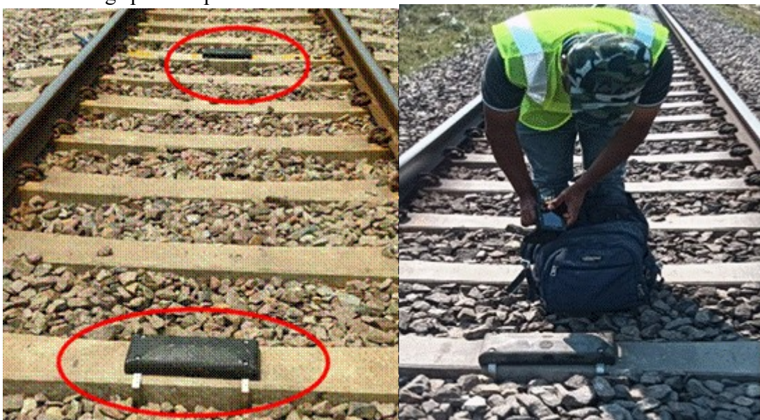
(Installation of RFID Tags on tracks)
