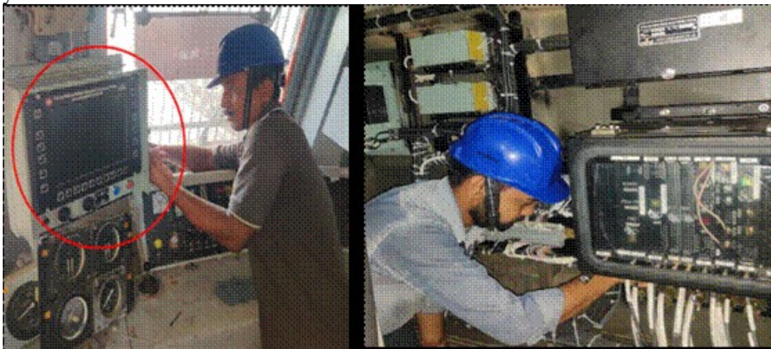
(Installation of Loco Kavach)
