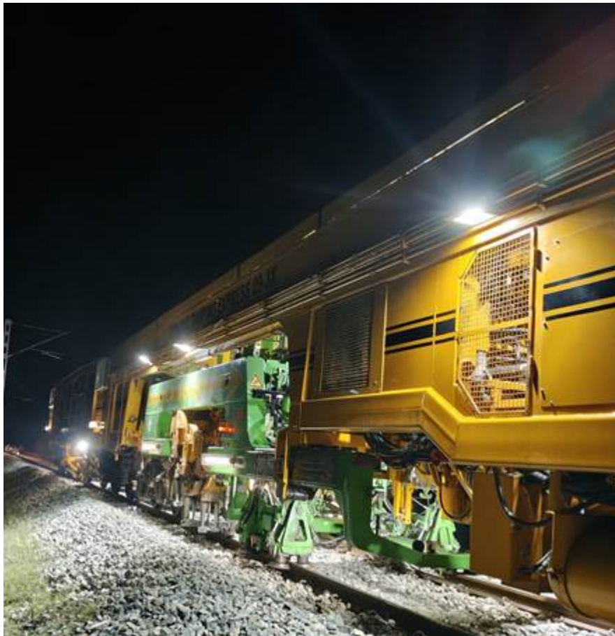
(Tamping machine working in valley section)
