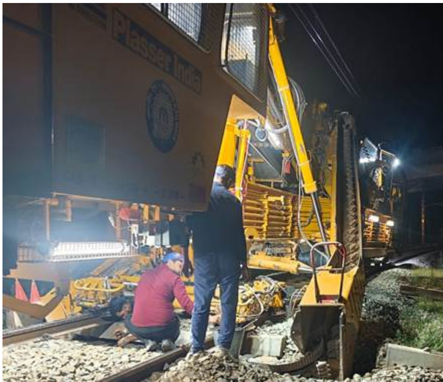
(Ballast Cleaning Machine working in valley section)
