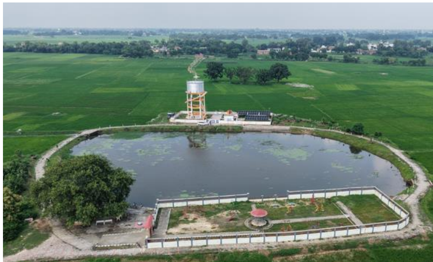
Water Supply Scheme at Sant Kabir Nagar
