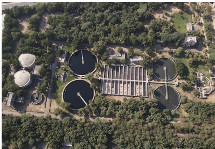
50.00 MLD STP at Salawas, Jodhpur
