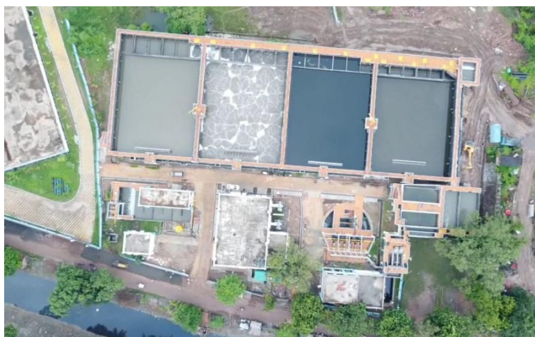
35.00 MLD STP at Maheshthala, Kolkata
