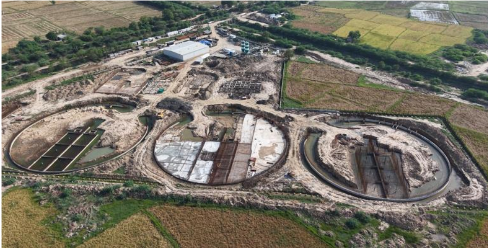
107.00 MLD STP at Ahmedabad, Gujarat
