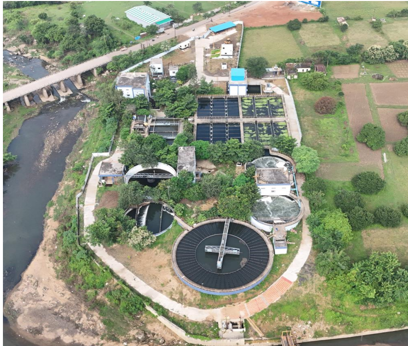
50.00 MLD Reuse at Chandrapur
