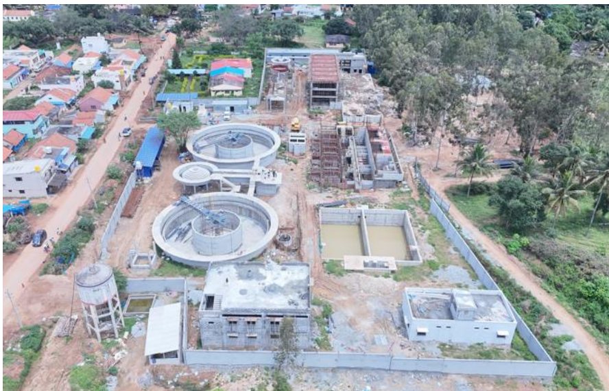
17.70 MLD WTP at Hassan, Karnataka
