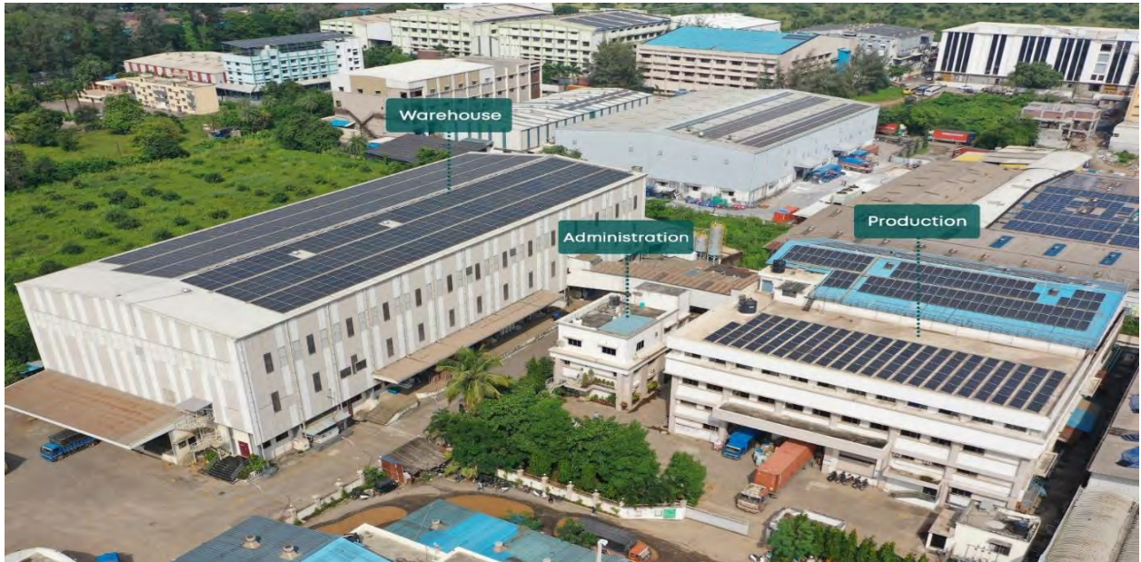
Above: photo of the Daman Facility.
